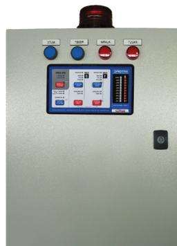
Level control system with MultiTrode® probe control
